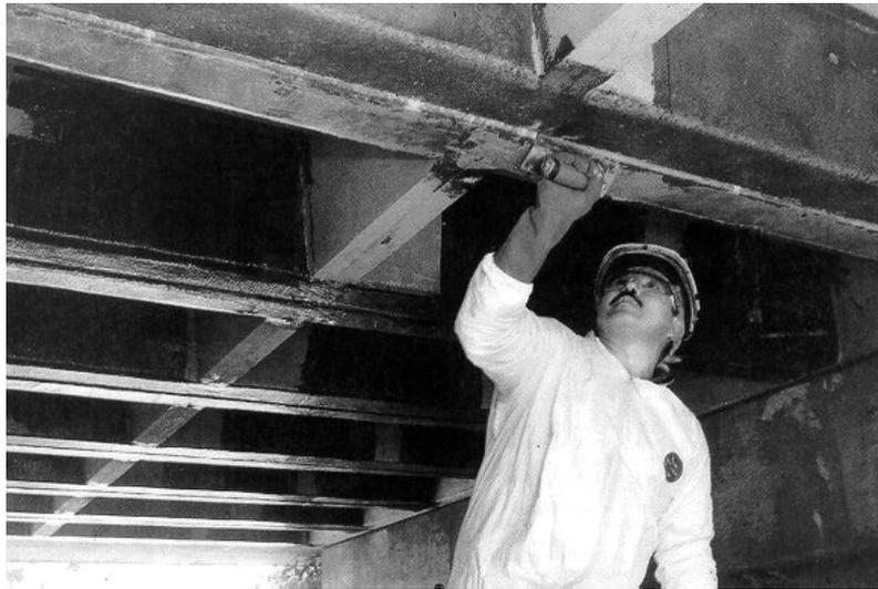
**Figure 3.** Application of FRP Reinforcement
