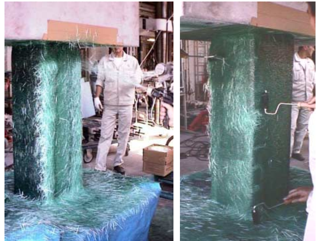
Photo 1. Construction site of sprayed-up FRP
