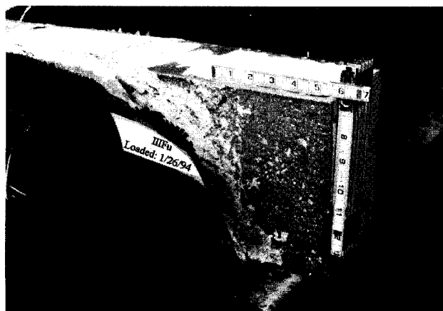
FIG. 11. Beam IIIFu: (a) Load versus CFRP Strain at Web; (b) Load versus Deflection; (c) at Failure
