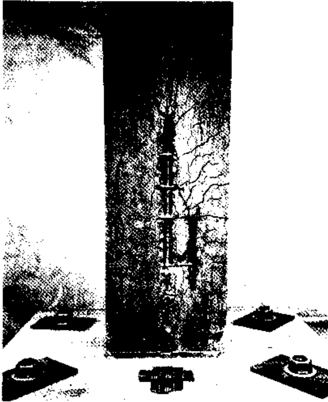
Figure 14. Shear cracks and failure of column R-3.
