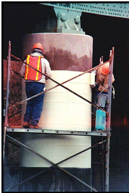
Aquawrap 22-77 Structural Prepreg Application
