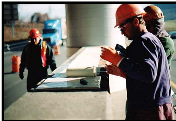
Laying-up Durability Samples
