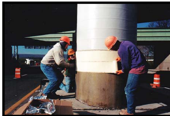
Structural Layer over Adhesive
