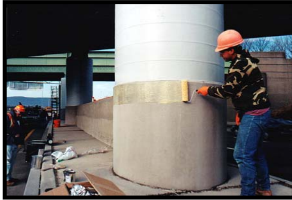
Roller Application of Adhesive
