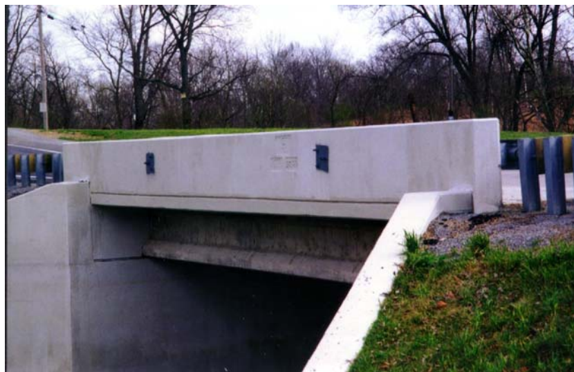
Figure 1. Roger's Creek Bridge - Bourbon County, Kentucky, USA
