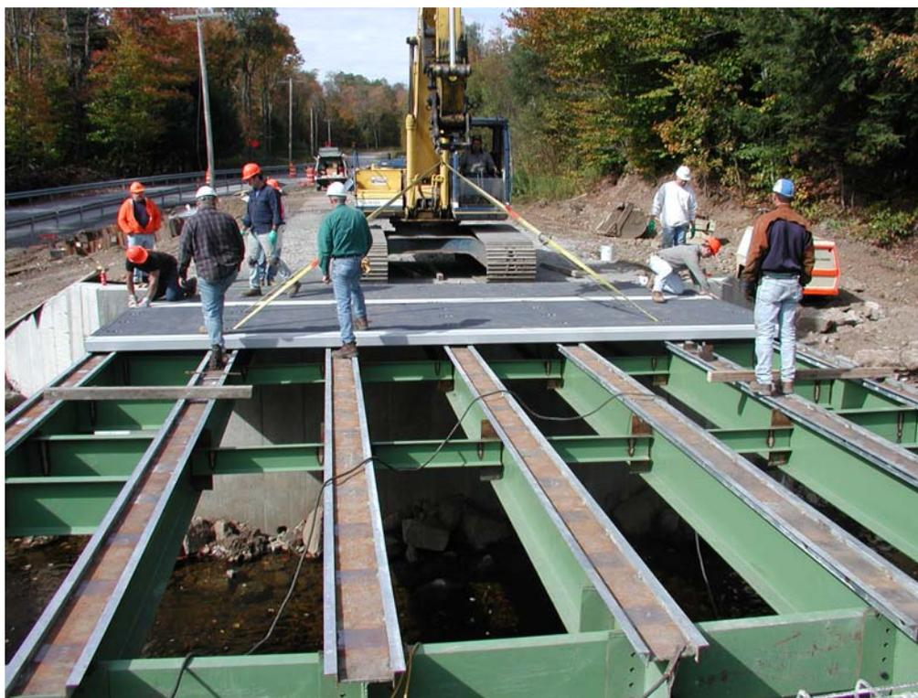
**Figure 12.** Five-Inch Deck Panels Being Installed on the Lewis County, New York, Bridge; October 2001.
