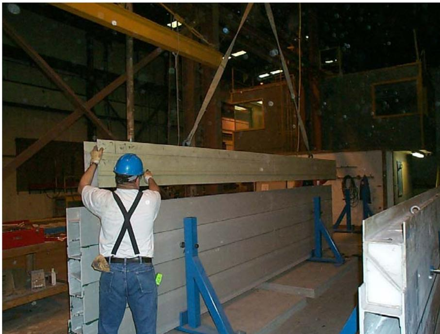
**Figure 11.** Bonding Deck Tubes to Make Panels for the Bridge Installation.
