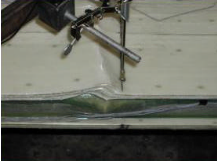
Figure 13. Buckling of Plate in Deck F10
