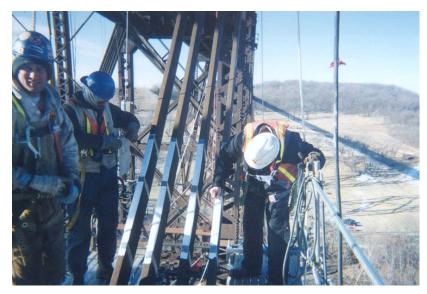
Figure 8-13 Manually Investigating the Tightness of Eyebars in Steel Bridges
