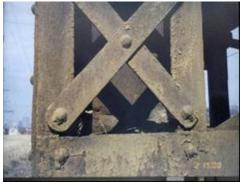
a) Bridge Structure b) Close-Up View Column Figure 5-1 Typical Built-up Steel Column of Steel Railway Bridge
