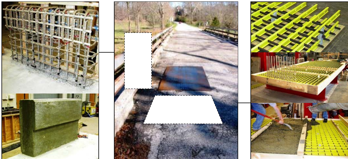
Figure 1 - Overview of FRP reinforcement systems for concrete deck and rail of new Bridge 1480230, Greene County, MO
