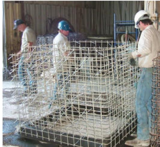
**Fig. 4: GFRP reinforcement cage**
