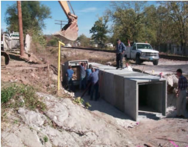
**Fig. 3: Installing of concrete box units**
