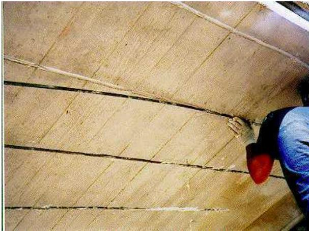
**Fig. 1: NSM FRP rods on deck soffit**
