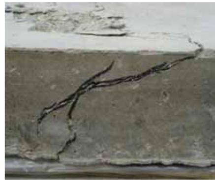
b) Shear crack along the support side
