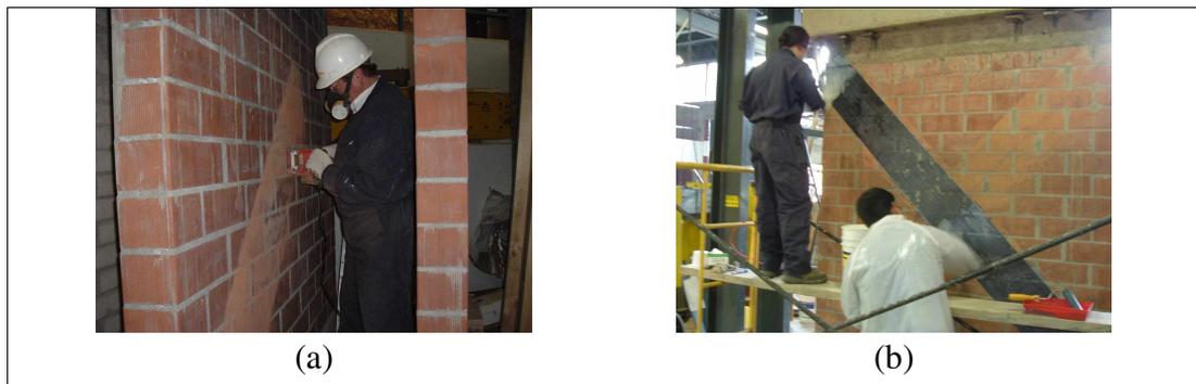
Figure 1. (a) Surface treatment of the walls. (b) Bonding of the FRP reinforcement.
