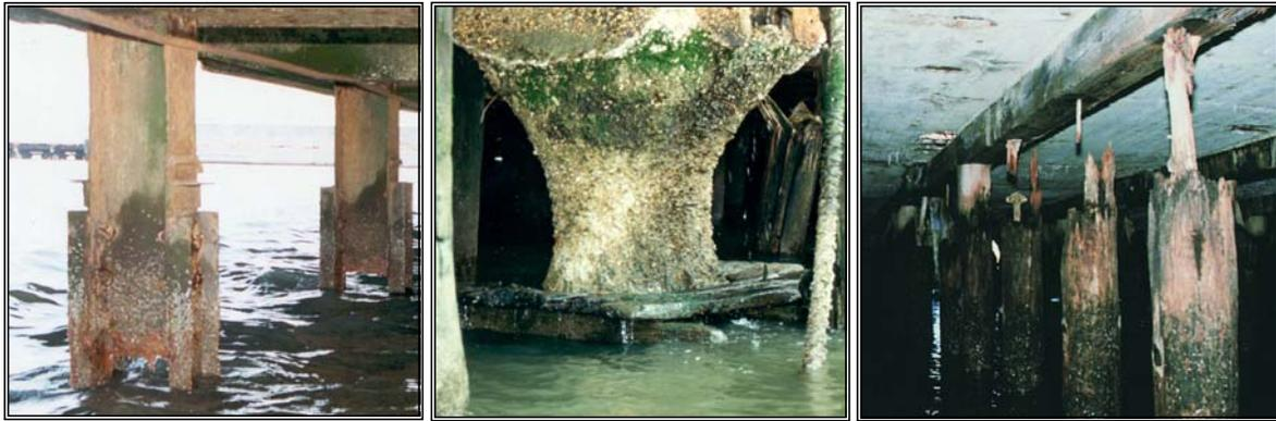
a) Corroded steel piles      b) Degraded concrete pile      c) Deteriorated timber piles
