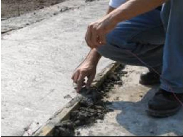
a) Installation of Thermocouplers
