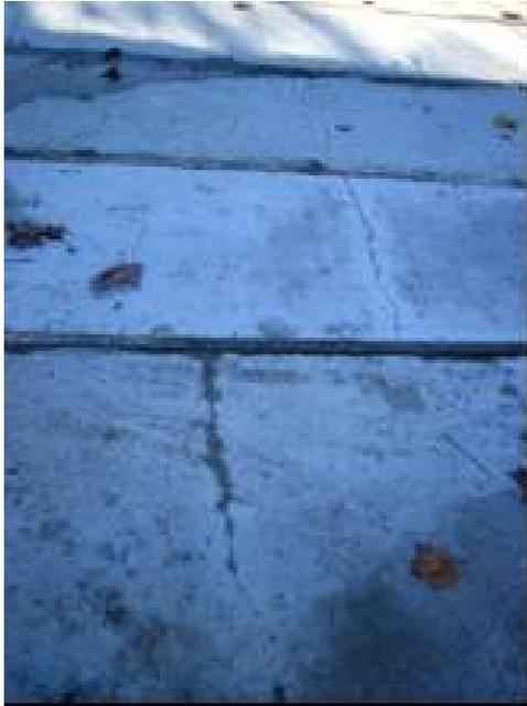
a) Transversal Cracks in Slabs
