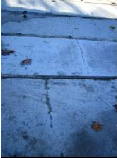
a) Transversal Cracks in Slabs
