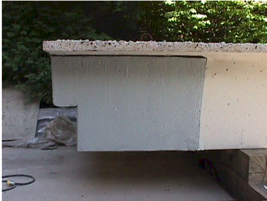
Step 1: Apply the Putty to Level The Concrete Surface and to Patch the Small Holes.
