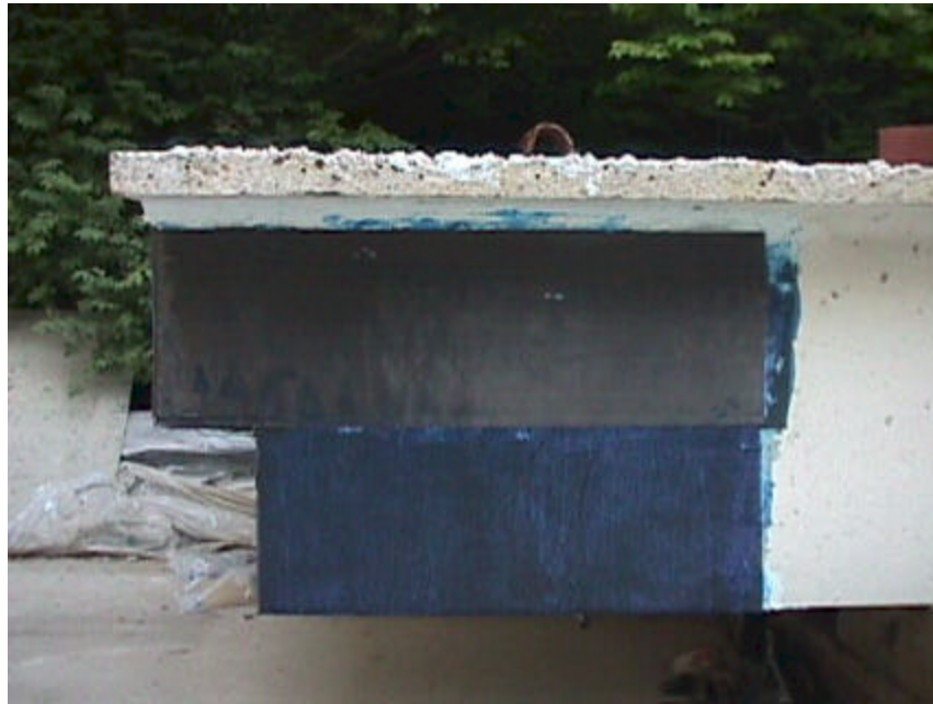
Step 7: Install Second Ply of 0^\circ U-Wrap of Laminate as Flexure and Axial Tension Reinforcement.
