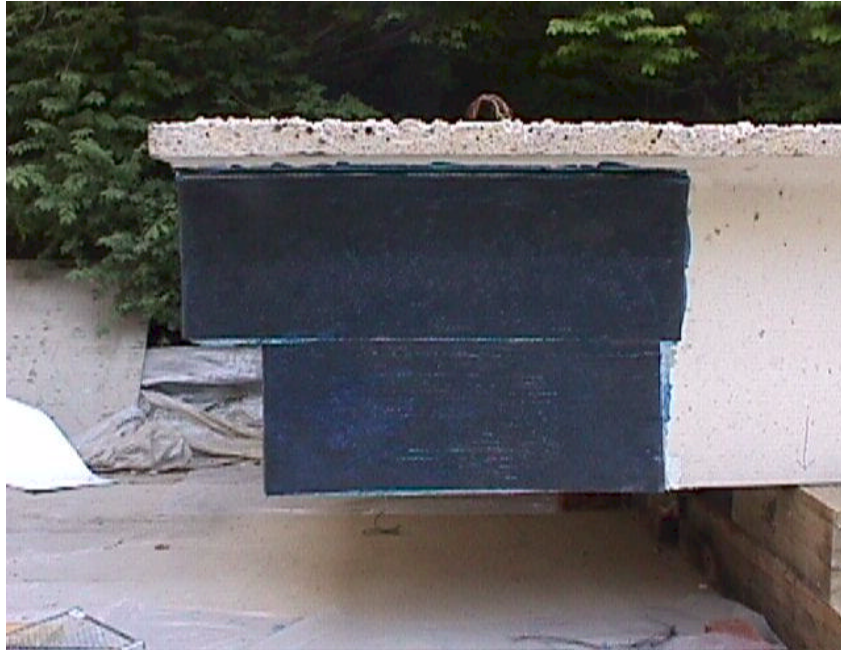
Step 3: Apply the Saturant to the Undapped Portion and Install 0° U-Wrap of Laminate for Anchorage of Reinforcement.
