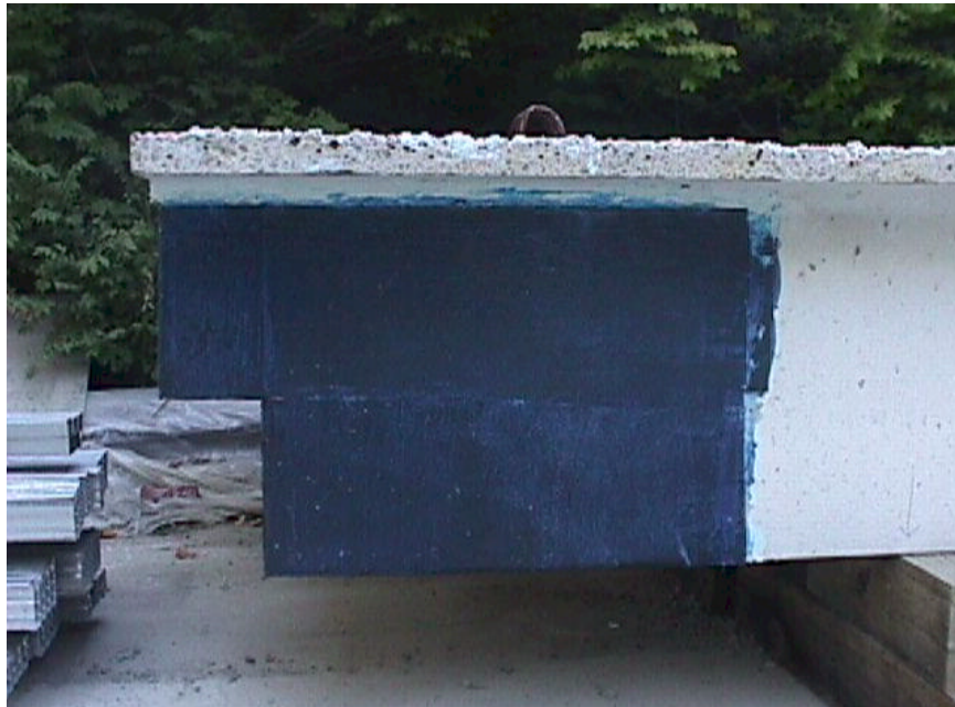
Step 8: Install Second Ply of 90^\circ U-Wrap of Laminate to the Extended End.
