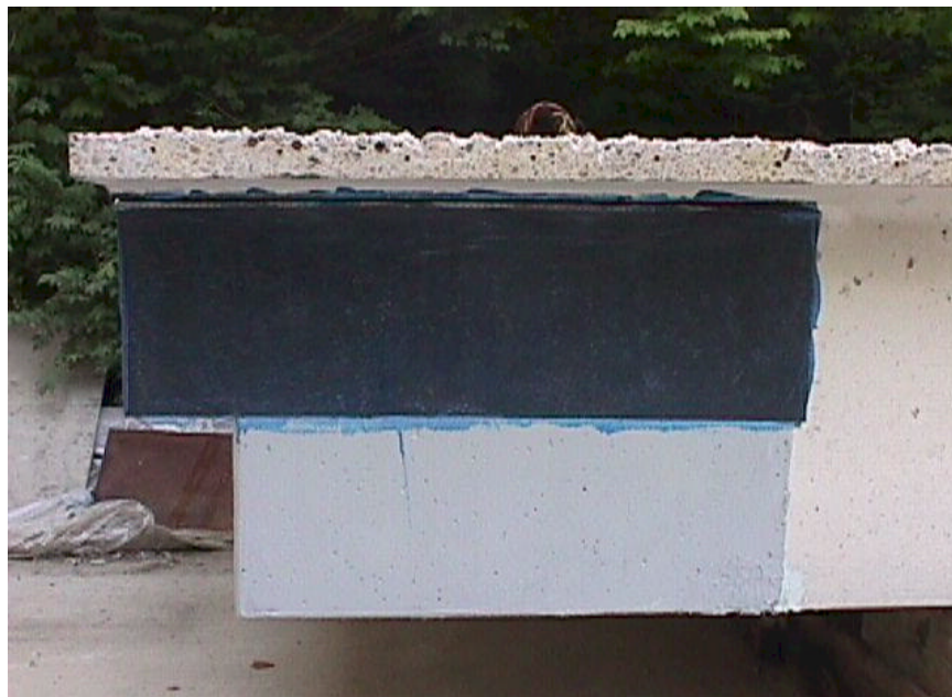
Step 2: Apply the Saturant and Install 0° U-Wrap of Laminates for the Flexure and Axial Tension.
