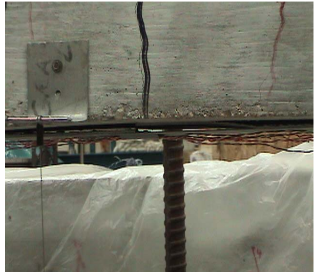
(b) Premature peeling in Beam 4
