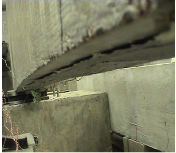
(f) Beam 6 after failure
