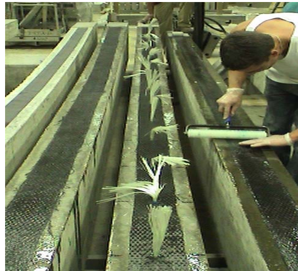
(b) Application of CFRP System
