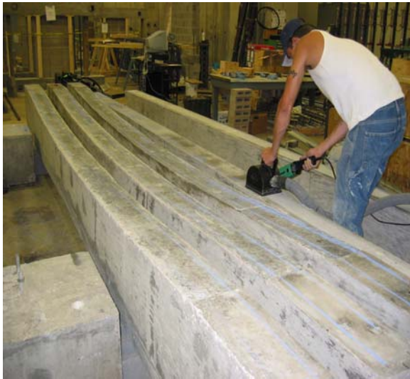
(a) Surface preparation before strengthening
