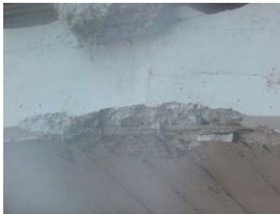
Figure 3-3. Reinforcement Exposed in the Bridge Crown
