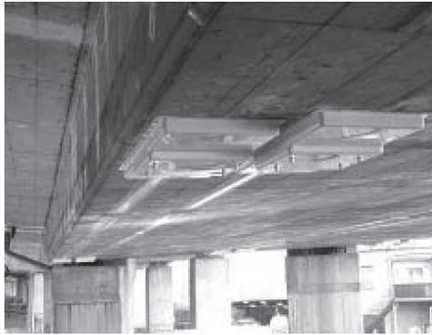
Photograph 2—Applied tensioned CFRP strip
