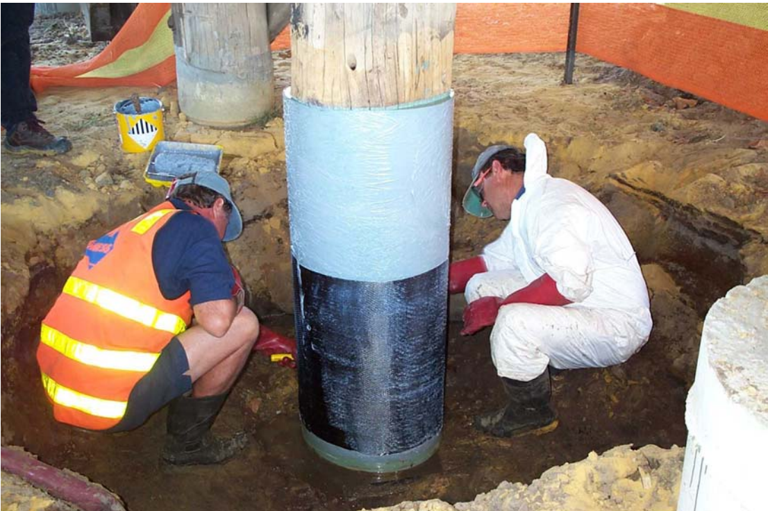
Narros Bridge Perth – FRP wrapping around columns (Photo)
