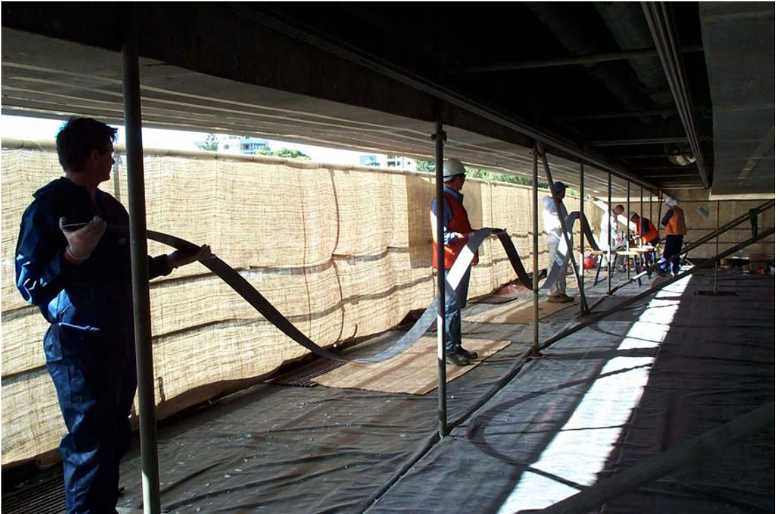
Westfield shopping center retrofitting work in progress (Photo)
