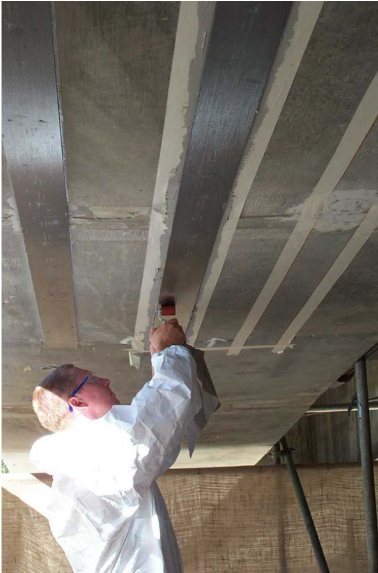
Oberriet – Meiningen Bridge deck retrofitting in progress (Photo)
