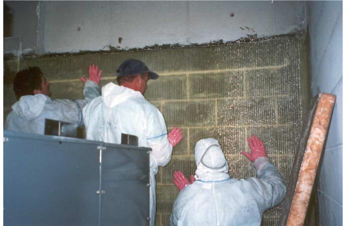
Contractor Richdale Builders Ltd engaged Contech to carry out seismic strengthening of the Milton and McFadden Street Substations using FRP composite materials. As both structures are of concrete block construction, consultants Sinclair Knight Merz (Wellington) designed a system that targeted specific wall areas to strengthen, and thus ensuring the survival, of these important structures in the event of an earthquake.
