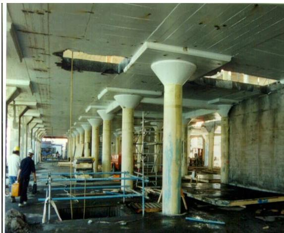
FRP composite wrapping was applied to more than 1,000 columns, after extensive concrete repair had been carried out to the columns and beams.
