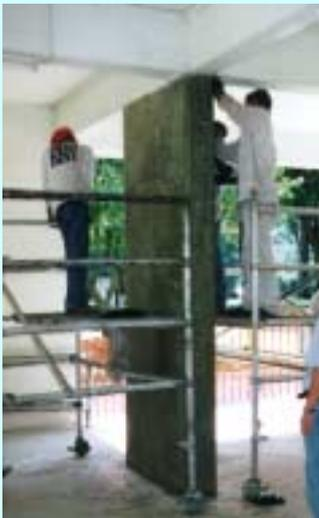
Axial load enhancement of a oblong column using GFRP
