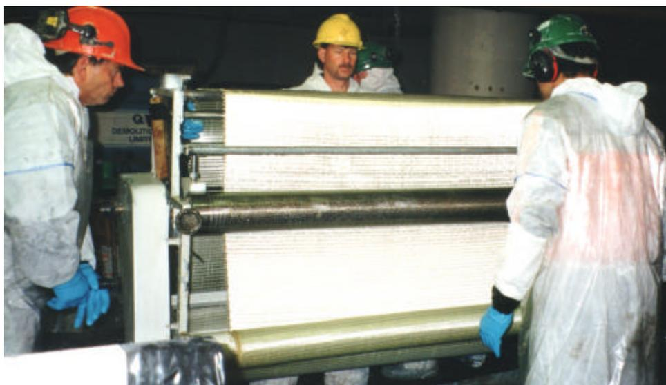
Fig 5.1: Impregnation of BBR GFS Sheet using a saturator
