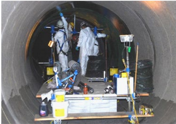
Application of tack coat on upper half of pipe.
