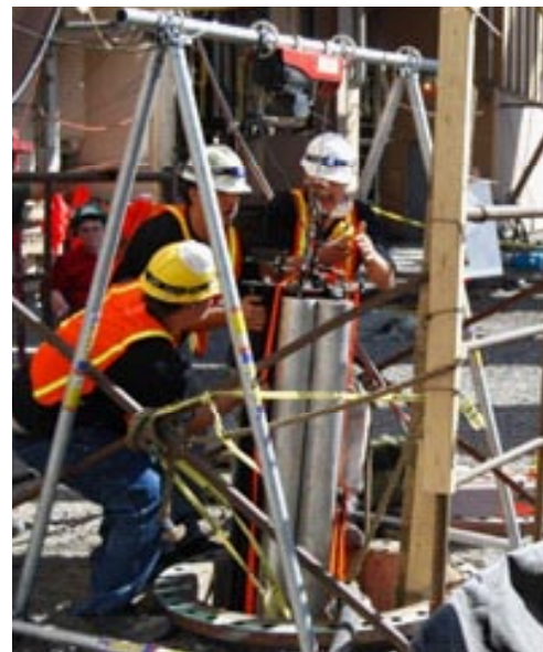
Equipment lowered through an existing manhole as the lining process begins.
