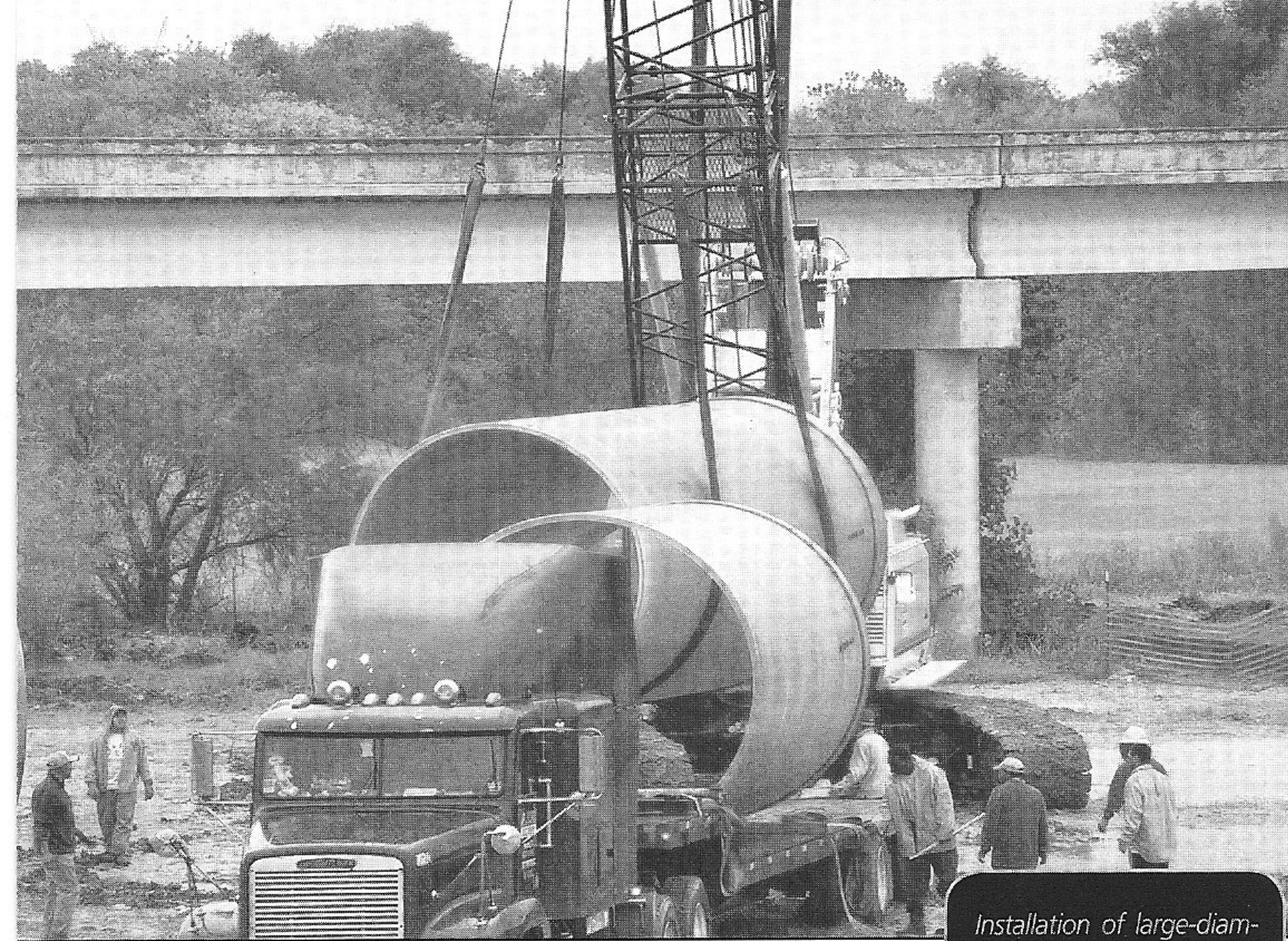
photo courtesy of Hobas Pipe
