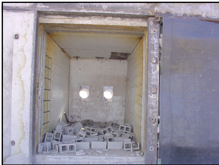
Figure 7: Un-retrofitted and CFRP retrofitted URM walls after the blast test
