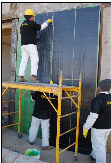
Figure 1: CFRP fabric installation on URM wall
