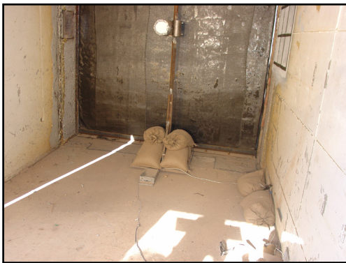
Figure 3: Instrumentation on the interior of the reaction building room
